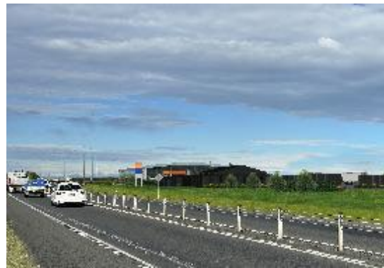
From SH2 Road looking west
