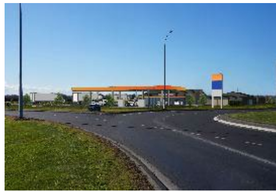
SH2 Road looking Northeast
