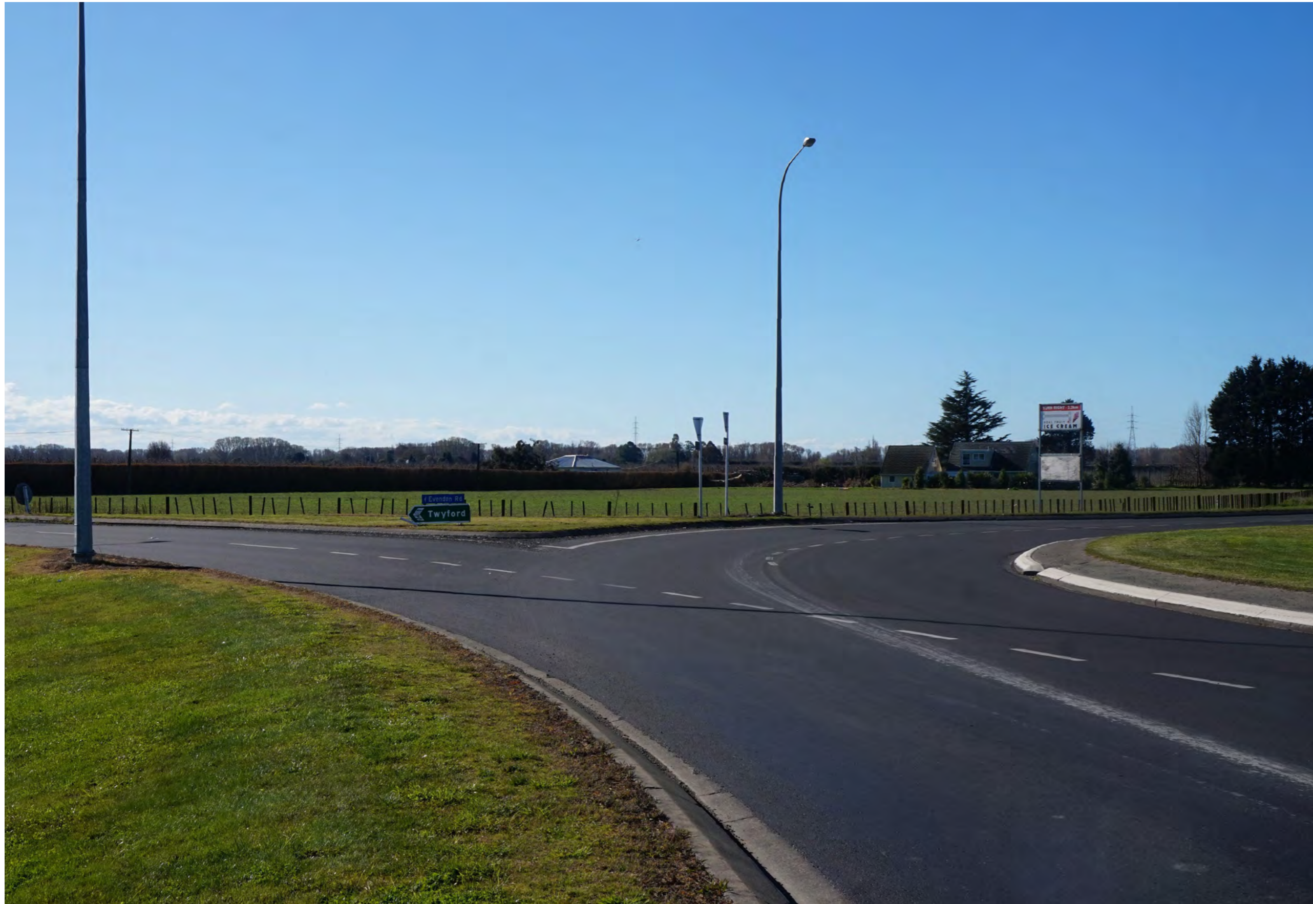
Photo 01 (09815): Image taken from SH2 Road looking Northeast
