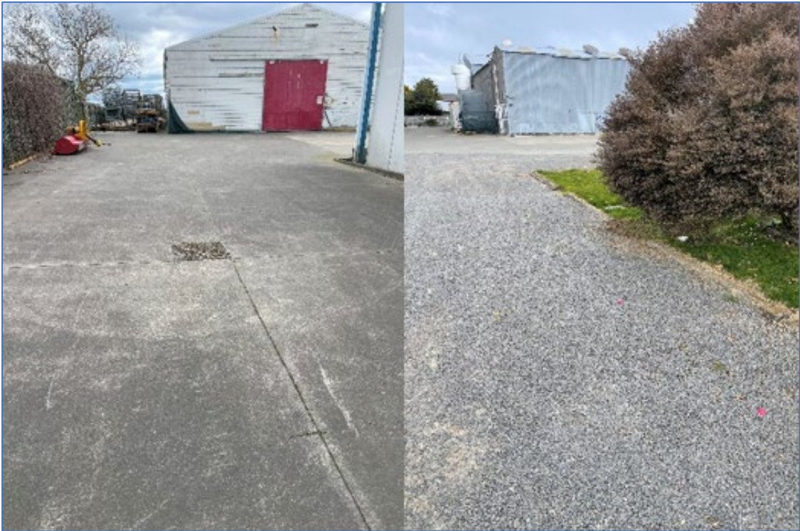
FIGURE 2: EXAMPLES OF SITE CONDITIONS.
