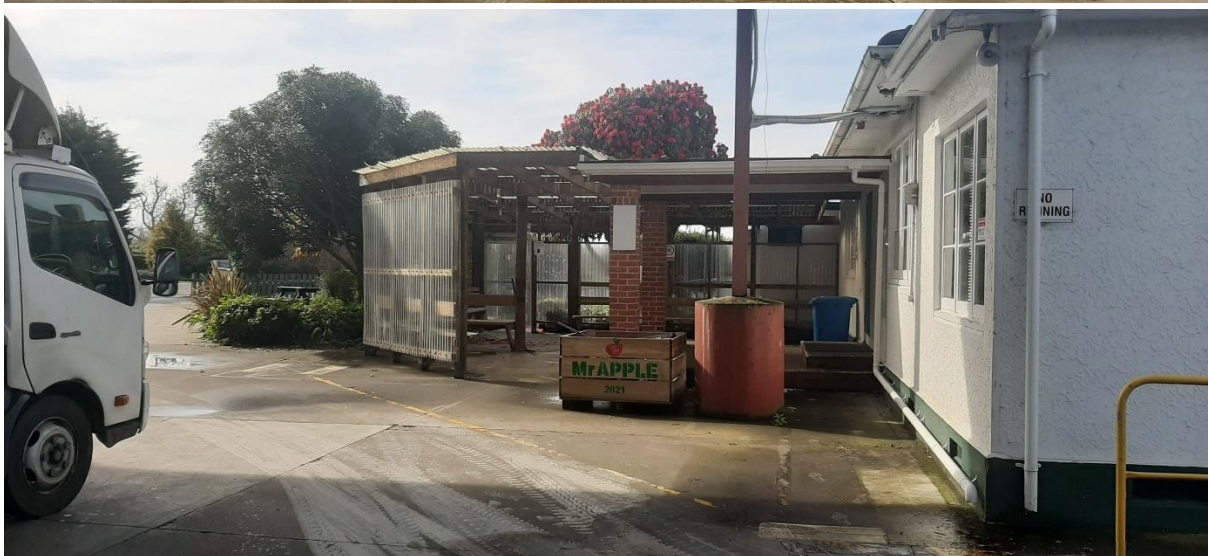
Top. Cool store on south-eastern corner. Middle. Sheds. Bottom. Office, lunch area
