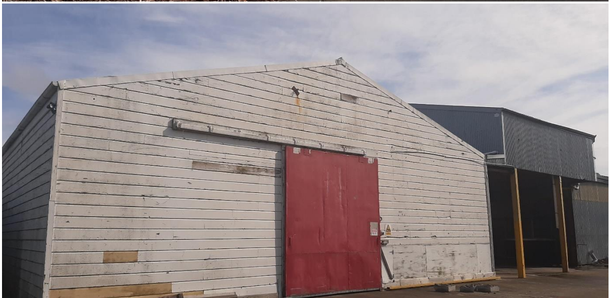
Above. Sheds on north-western boundary
